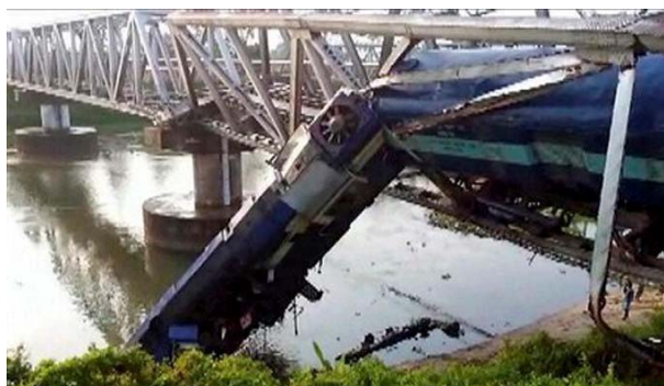
Fig 1: Accident occurred due to track breakaged.
